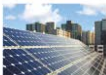
光伏逆变 Photovoltaic inverter
